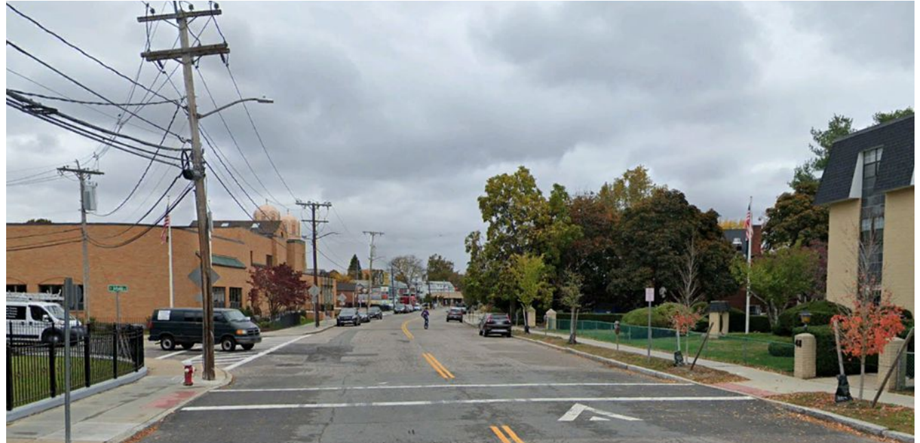
Raised Crosswalk at Bigelow Avenue, Watertown
