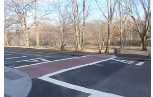
Raised Crosswalk at Pond Avenue, Brookline
