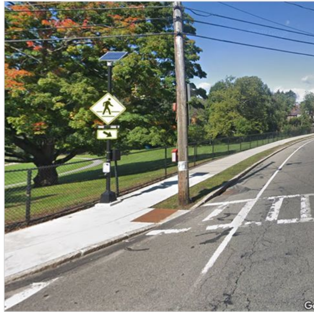
RRFB at Warren Street, Chestnut Hill
