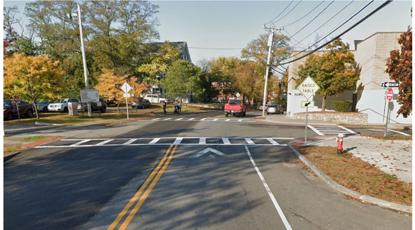
Speed table at Nichols/Elton Avenue, Watertown Specified by VAI, installed in 2016
