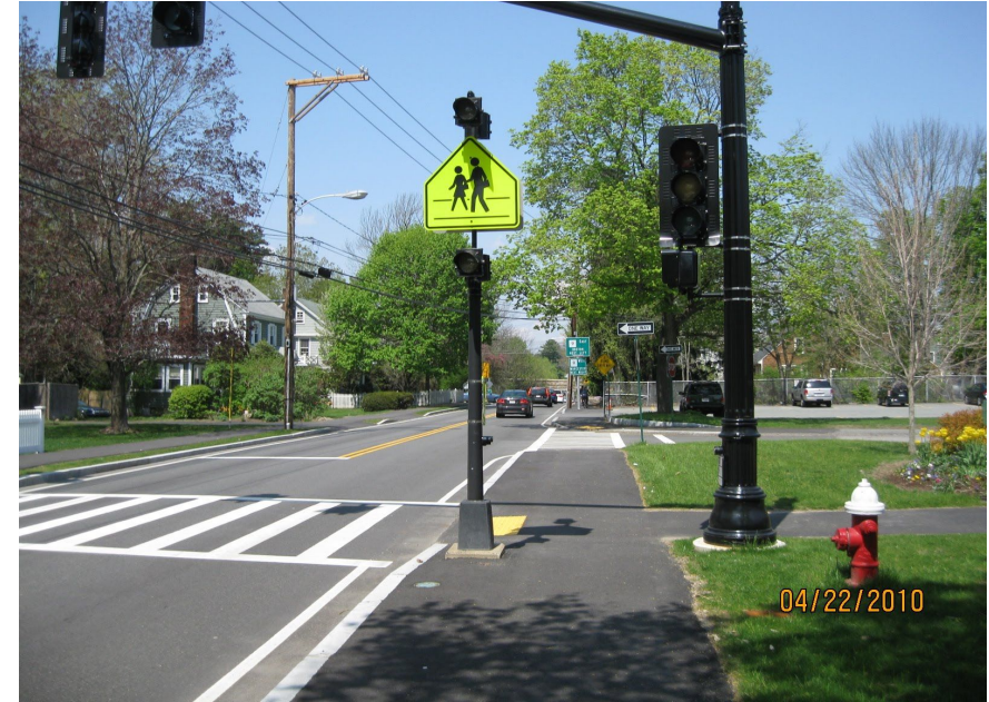
RRFB at Weston Road, Wellesley
