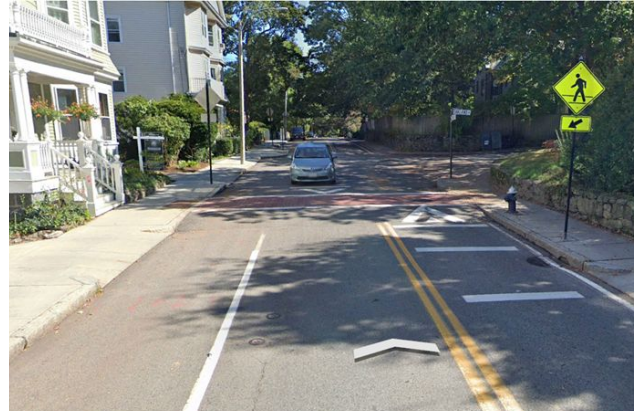
Raised Crosswalk at Walnut Street, Brookline
